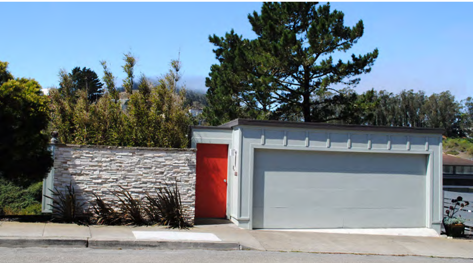
[6-22] (top) 72 Turquoise Way, Hayes & Smith, Galli Construction Co., 1964. [Hannah Simonson]
