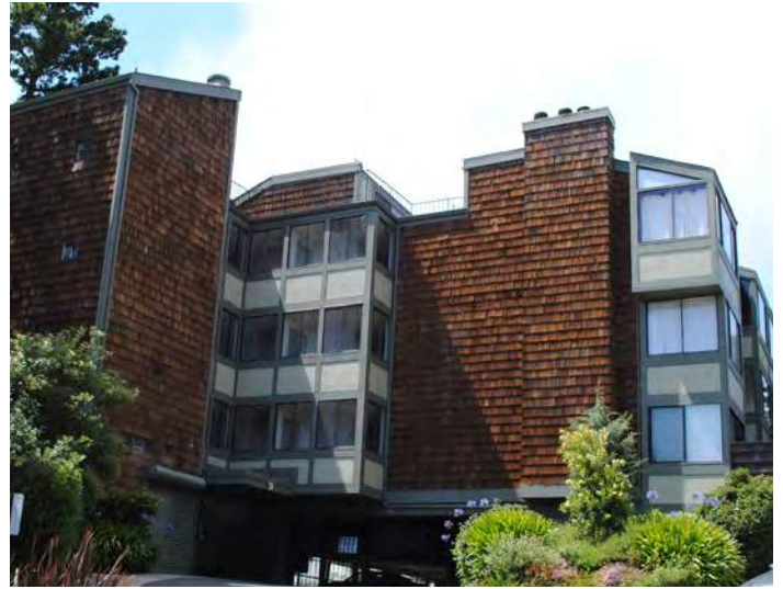
[5-12] Gold Mine Hill Apartments, 43 Ora Way | This apartment complex retains an exceptionally high degree of integrity. The painted green panels under the windows, were originally red, all material details are original. [Hannah Simonson]
