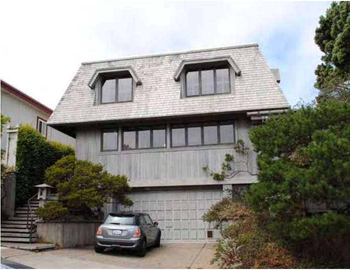
[5-3] 66 Everson Street | This is a rare (for Diamond Heights) example of a custom, architect-designed Second Bay home. Designed by Charles Warren Callister, the house has extremely high integrity. [Hannah Simonson]
