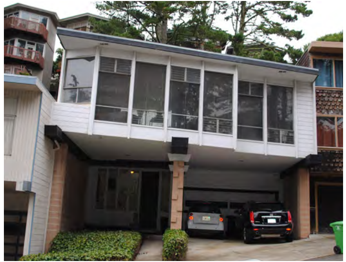
[5-8] 319 Amber Drive | This house designed by Harold Dow was part of a small, 3-house development. As the only fully intact example of the three, and for its distinct Mid-Century Modern features including original louvered aluminum frame windows, this resource may be eligible as an individual resource or as a district contributor. [Hannah Simonson]
