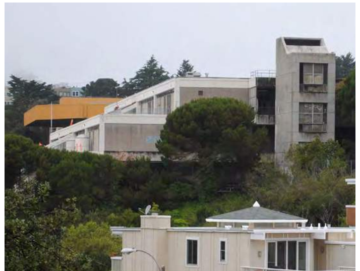
[5-17] SOTA High School, may be usefully understood as a Brutalist resource, but requires further investigation in order to determine character defining features and integrity (public access is restricted due to their current use). [Hannah Simonson]
