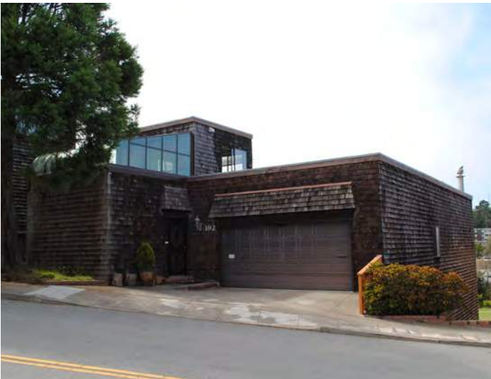
[5-13] 9 Jade Place | This home is one of a tract designed by John Baumann for Progressive Builders. Each of these houses has a unique design, but a cohesive Third Bay style. 9 Jade Place retains high material integrity. Wood single siding and the glass covered porch are character-defining details. [Hannah Simonson]
