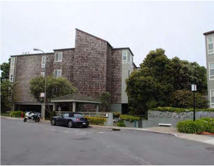
[5-11] Diamond Heights Village, 115 Red Rock Way | This complex designed by Joseph Esherick and Arthur Gensler is the work of two master architects in a new style, typified by the shingle siding and shed roofs. Windows have been updated, but in a compatible configuration and consistently throughout the complex. Landscape design is a key character-defining element. [Hannah Simonson]
