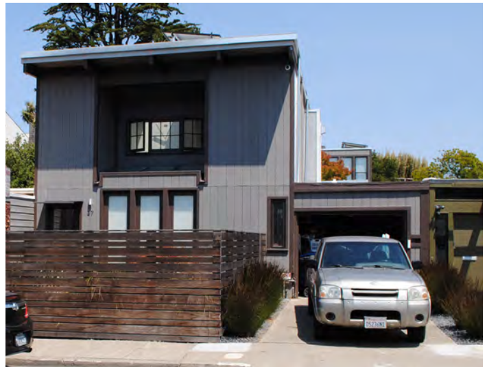
[5-10] 37 Cameo Way | This home would be considered a non-contributor due to loss of integrity. The original design of the Eichler homes on this block are extremely low-lying, single story houses. The prominent second story addition on this house destroys the character of this resource and diminishes the character of the surrounding resources by invading privacy and sight-lines. [Hannah Simonson]
