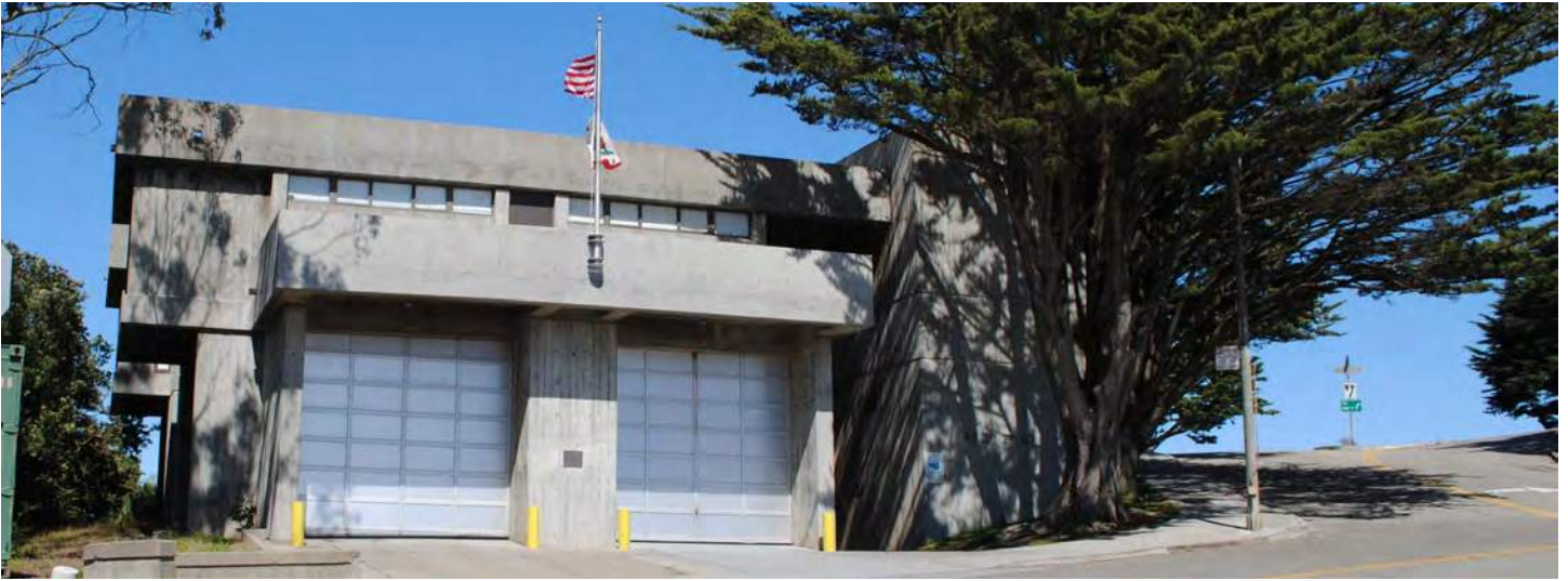
[5-15] 80 Digby Street | Fire Station No. 26 (formerly known as the John F. Shelley Fire Station) was designed by Rockrise & Watson with landscape design by Roysont, Hanamoto, Mayes & Beck. The building is a full expression of the character-defining tenets of Brutalism - including exposed, structural concrete with visible texture from wooden formwork, strong right angles, strong geometric massing, and recessed windows and openings that read as voids. This building has very high integrity and is potentially eligible as an individual resource under Criterion C/3. [Hannah Simonson]
