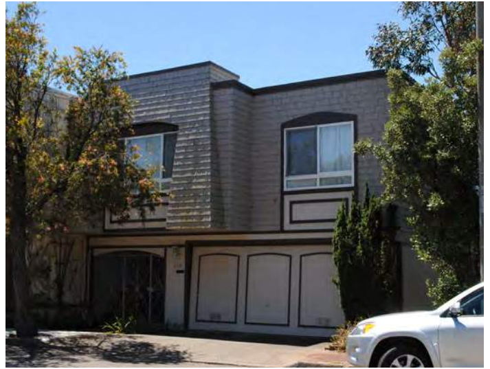
[5-22] 216 Gold Mine Drive | This Galli house retains its original shingles, siding, garage door, light fixture, and house numbers. It is relatively rare that these homes still have original garage doors. The windows, however, have been replaced. [Hannah Simonson]
