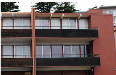
Repair & Maintain In Place
